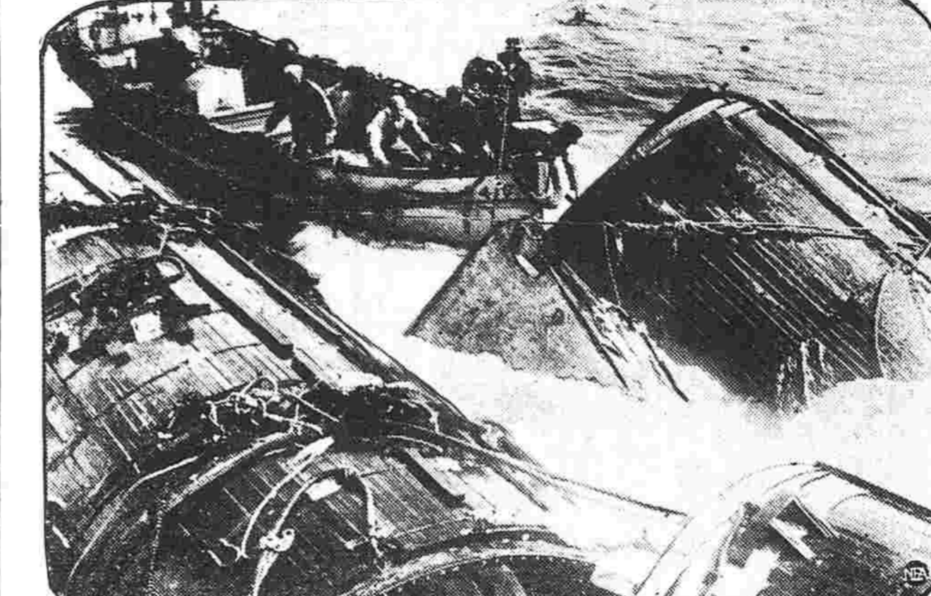
Giant pontoons had just raised the nose of the lost Navy submarine S-51 above the waters off Block Island, R. I., when—crack!—a cable snapped. Months of work by a gallant salvage corps went by the board as the heavy ship sank back to the ocean bed. The nose of the submarine can be seen in the center of the picture, supported by pontoons, an instant before the mishap.
